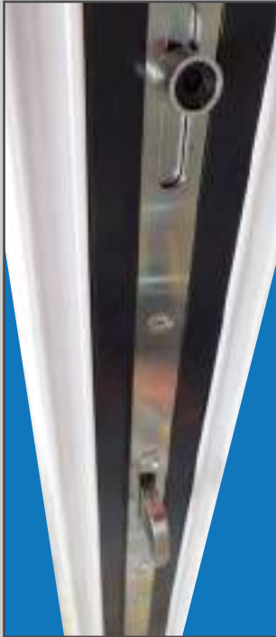
View of lower hook bolt and cam
